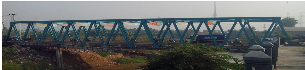
Fig. 2. Photo of Warren Truss Bridge.
