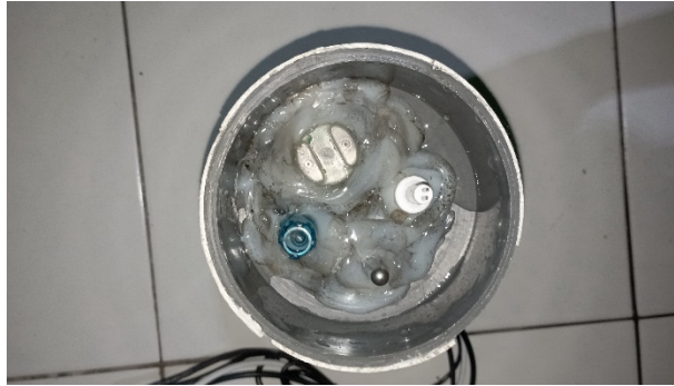
Fig. 8. Sensor Installation on Pipe
