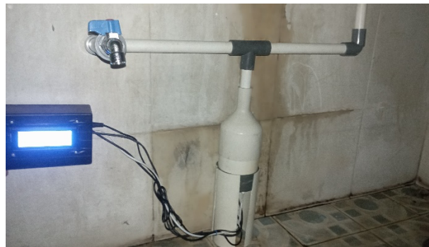
Fig. 9. Installation of Tools on Waterways
